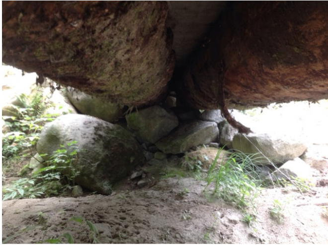
pedestrian bridge left abutment
