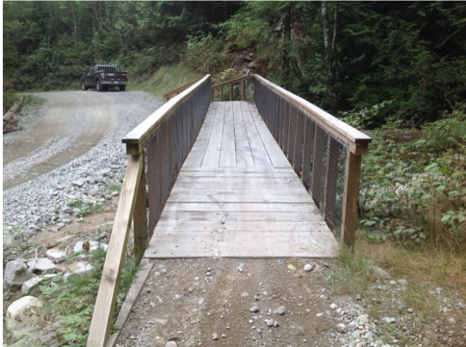
pedestrian bridge - left approach
