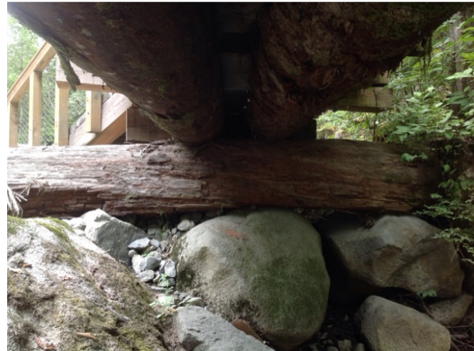
pedestrian bridge right abutment
